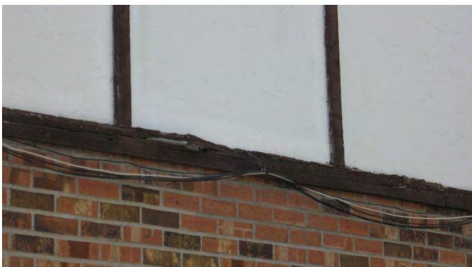
Parcel #19: Exterior wiring; portions of façade in poor condition.
