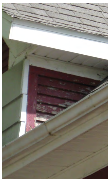
Parcel #3: Peeling paint; exposed wood; faded paint/patch.
