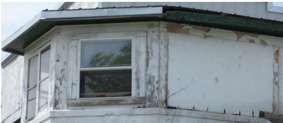
Parcel #20: Peeling paint/exposed wood on door; cracked façade; broken glass window brick; boarded up window/door; windows in poor condition (3 pictures).
