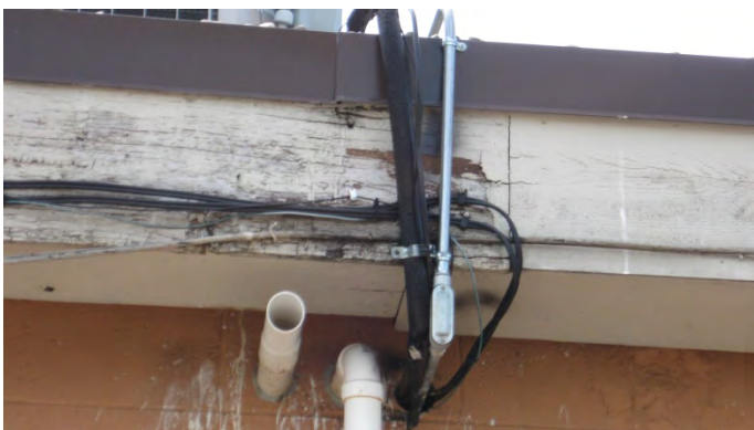
Parcels #10-16: Exterior wiring & exposed/rotting wood; peeling paint.
