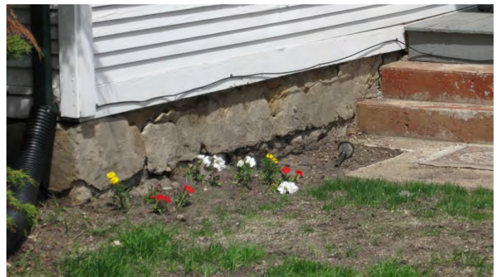
Parcel #5: Unimproved gravel driveway & outdoor storage of items; peeling paint and exposed wood; rotting porch, foundation in poor condition.
