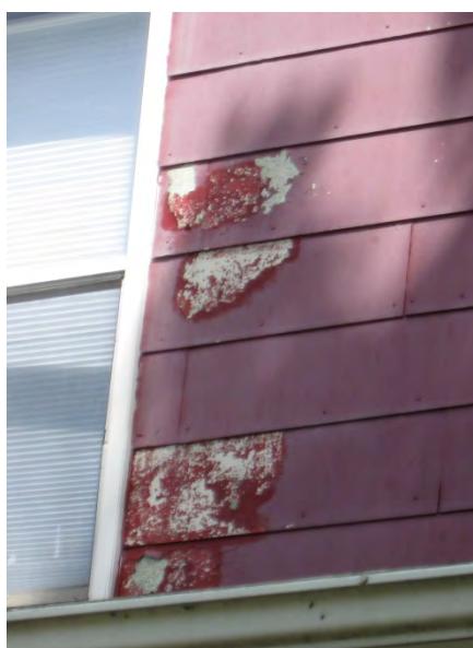
Parcel #3: Peeling paint; exposed wood; faded paint/patch.
