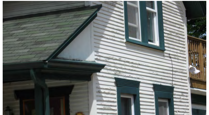
Parcel #4: Peeling paint & exposed wood on garage; rotting wood at front door; rusted siding nails & foam sealant at window.
