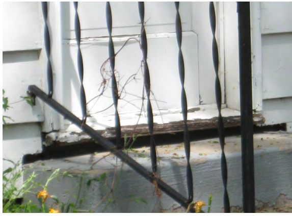
Parcel #4: Peeling paint & exposed wood on garage; rotting wood at front door; rusted siding nails & foam sealant at window.
