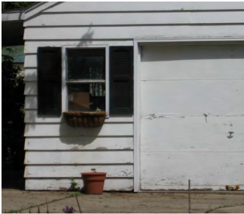
Parcel #4: Peeling paint & exposed wood on garage; rotting wood at front door; rusted siding nails & foam sealant at window.
